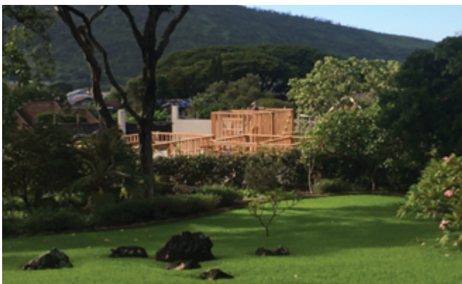
View of VEH construction from Hogan House, current MHC offices.
