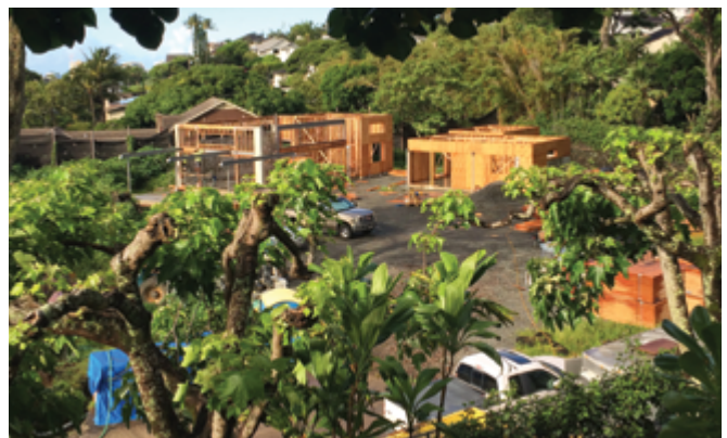
The walls are up on the Visitor Education Hale!
